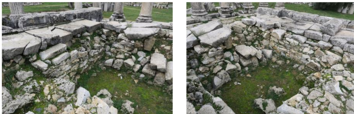
Figure 10-11: The wall of under the paving naos blocks
